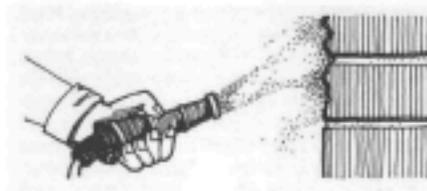
material. Another common type of cleaning is abrasive blasting. Water blasting, sodablasting, and sandblasting are techniques that should never be used to clean masonry surfaces. This damages and erodes the brick and mortar joints.
